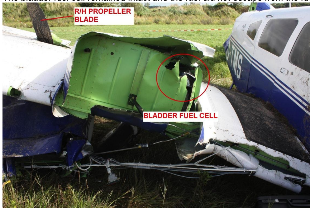
Figure 15: view of the right hand engine nacelle structure and fuel cell
